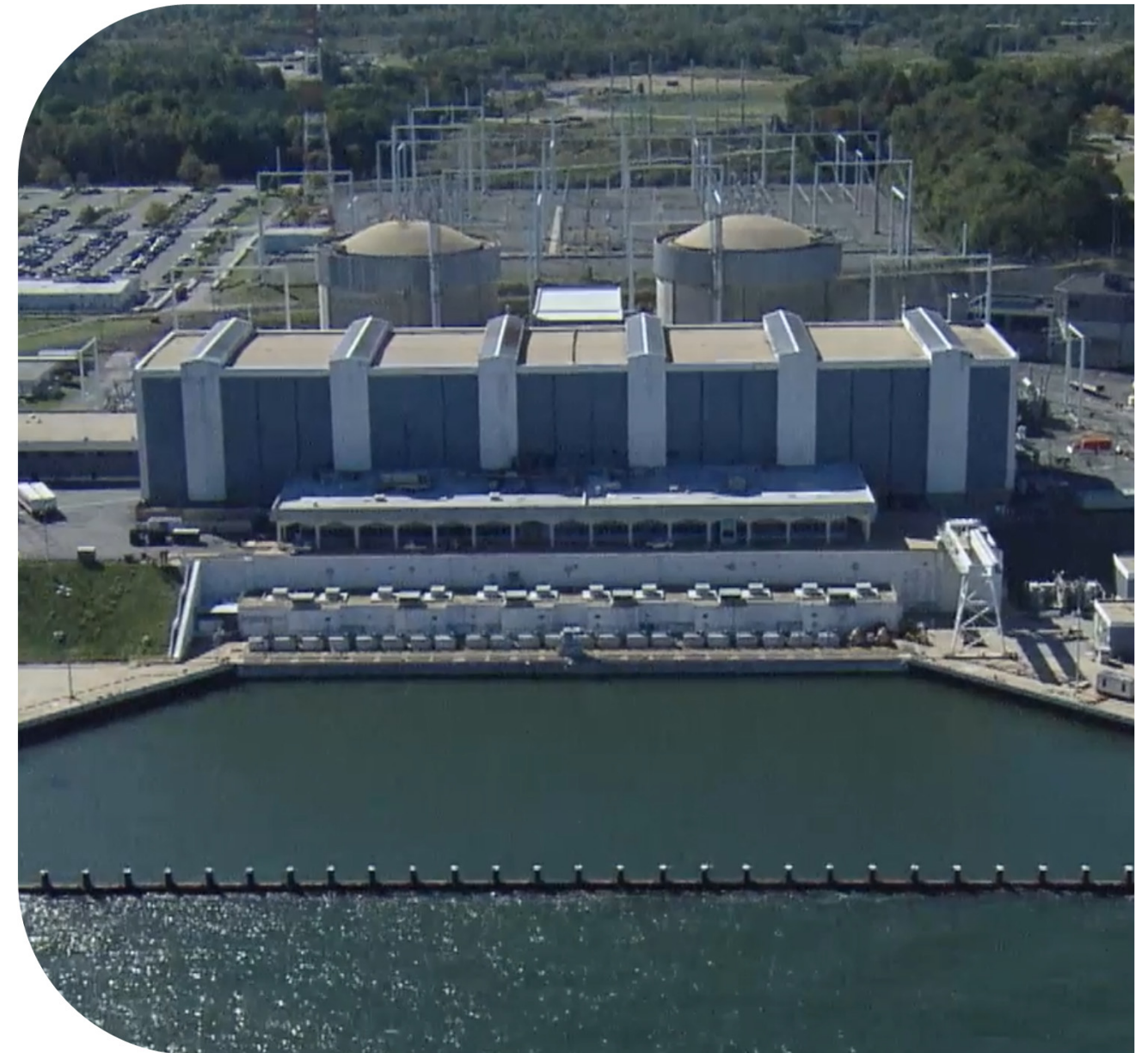
Calvert Cliffs Clean Energy Center
