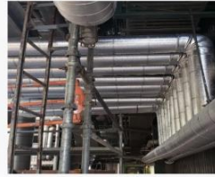
Enhanced Piping Insulation
