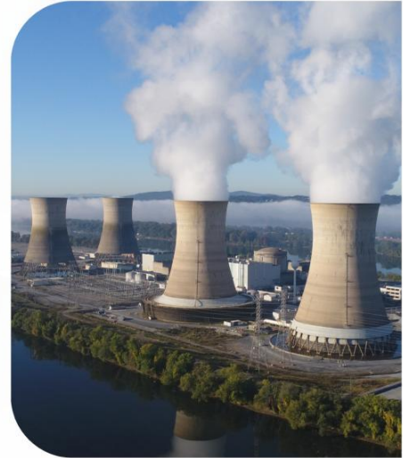
Crane Clean Energy Center
